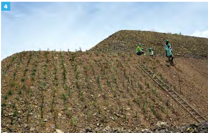
4 Planting after construction for slope protection
