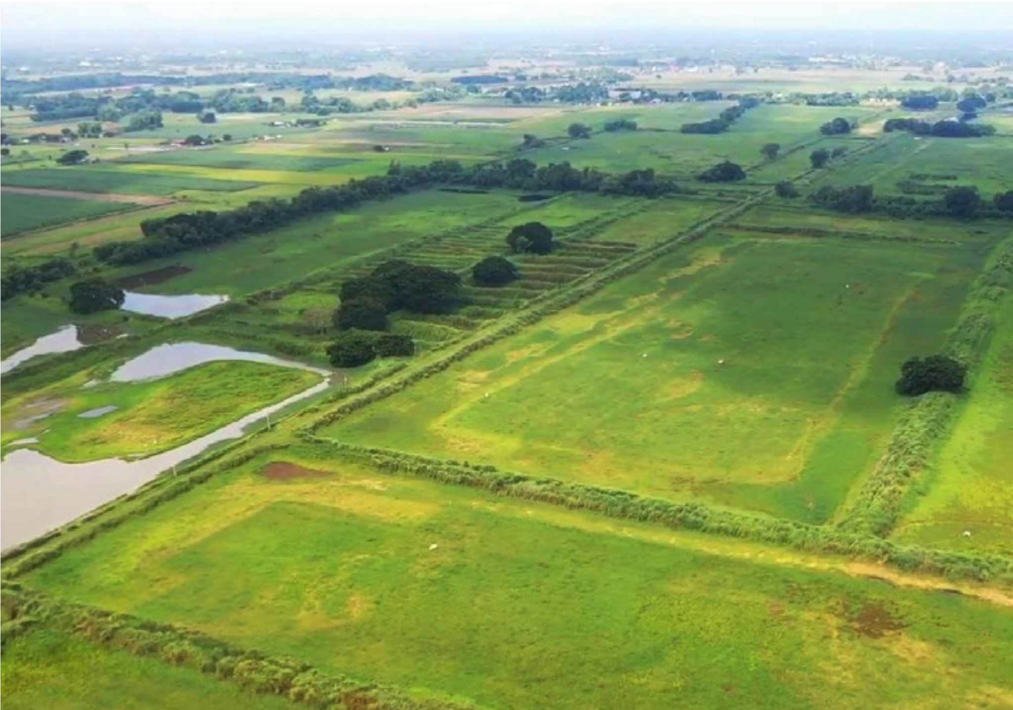
Site of the Liberty Floating Solar Project Phase A and B in Paniqui, Tarlac
