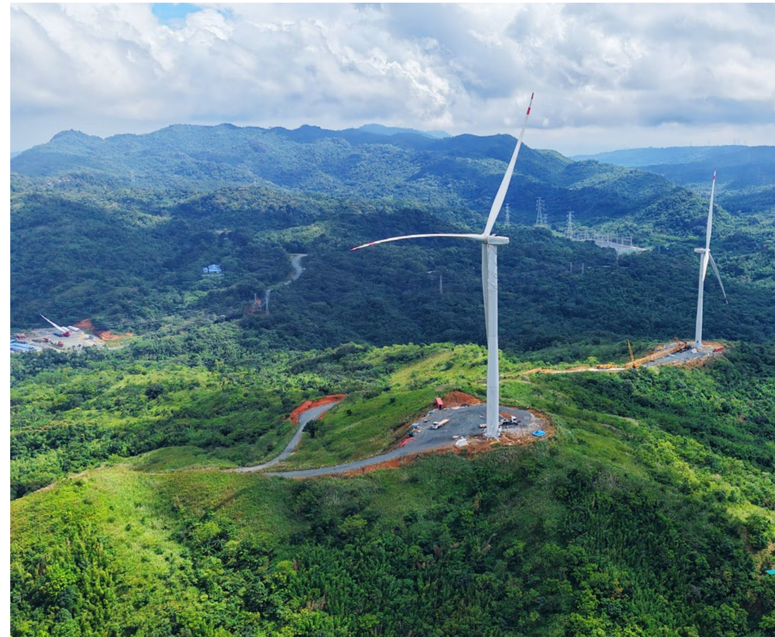
Tanay Wind Power Project completes installation of 2 WTGs
