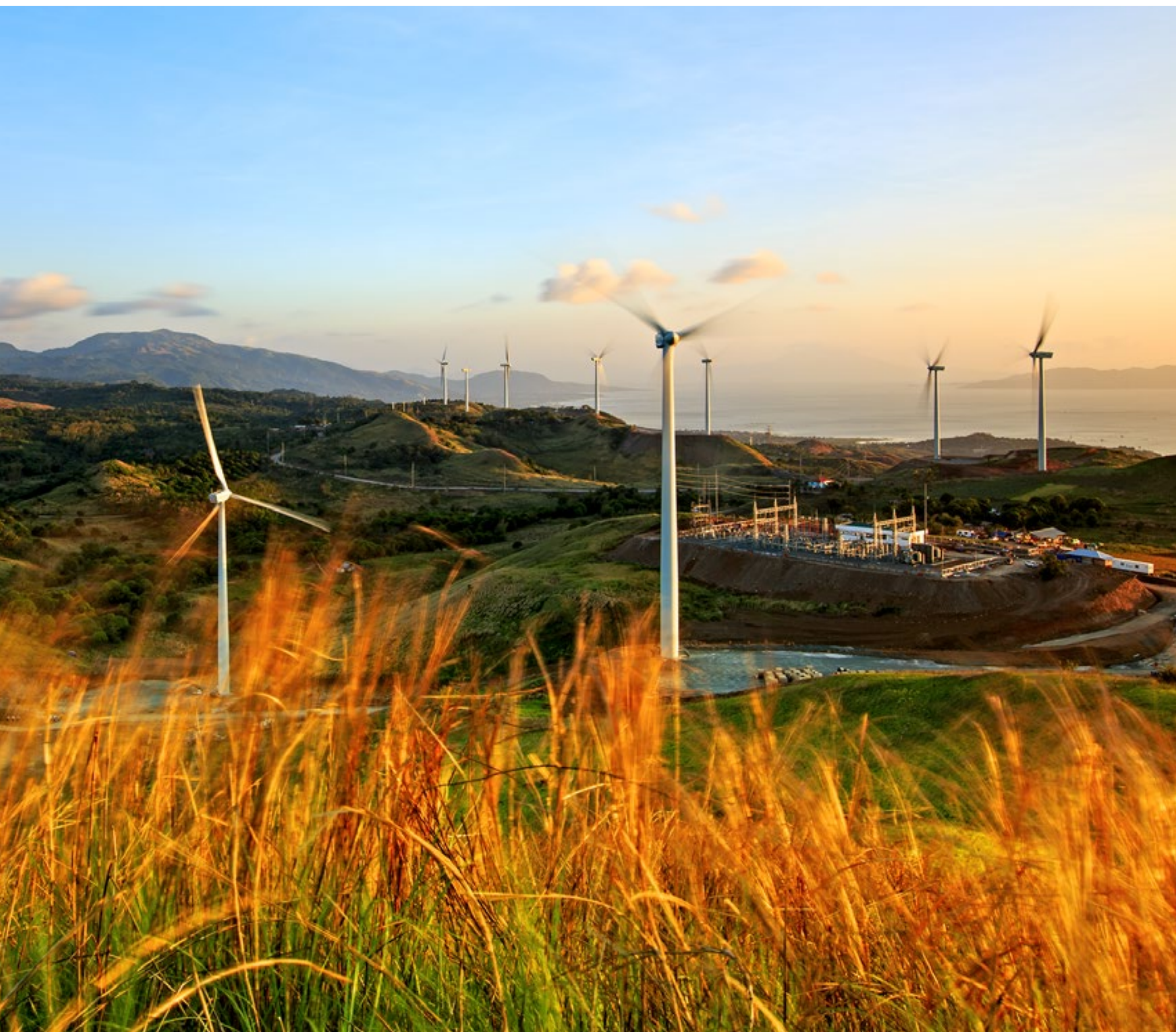
54 MW Pililla Wind Farm in Pililla, Rizal
